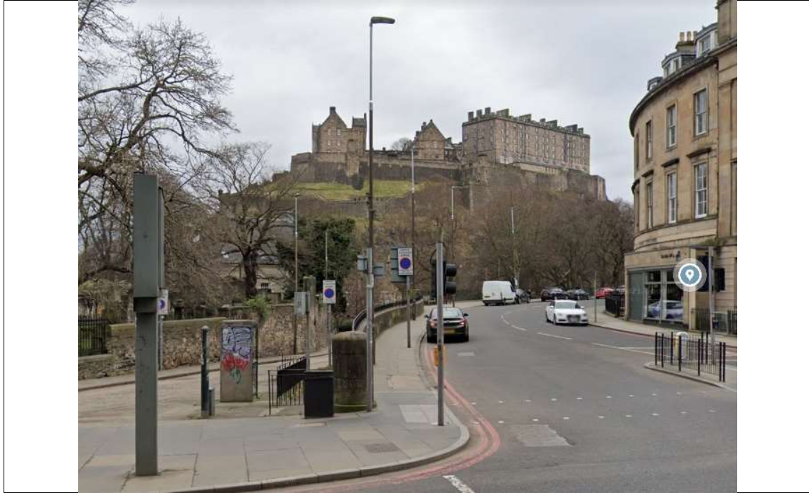
Image 4 – Existing payphone kiosk the junction of King's Staples Road to be replaced
